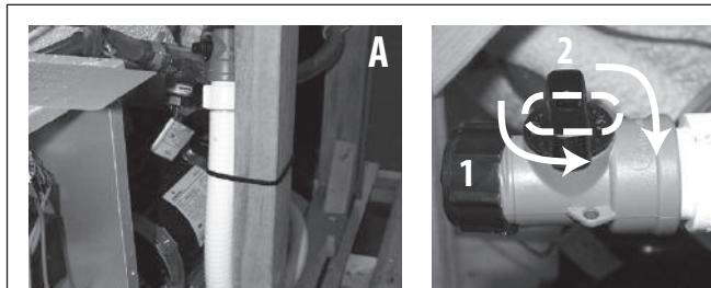
**4.** Place the drain pipe on the ground and unscrew the cap (1) to empty the water (away from the hot tub). If present, open the valve (2). DO NOT OVERTIGHTEN!
